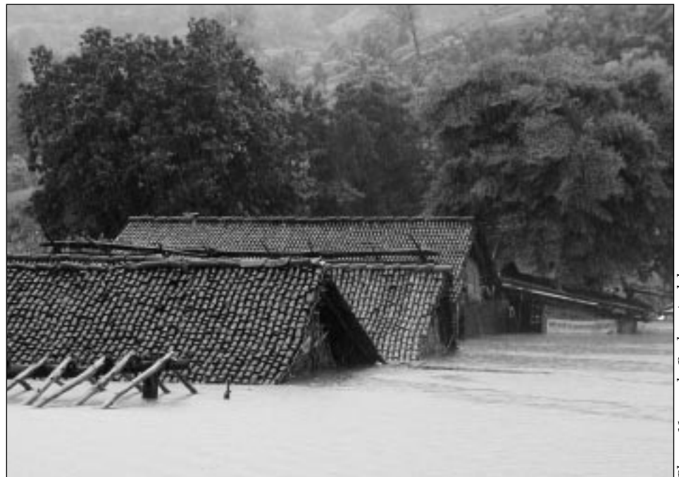
Houses submerged by Sardar Sarovar reservoir, India.
